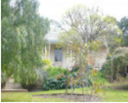
26 Mercer Street, Queenscliff
