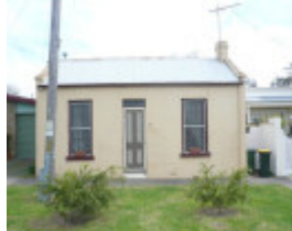
36 Mercer Street, Queenscliff
