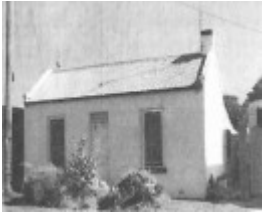
36 Mercer Street, Queenscliff
