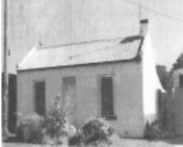
36 Mercer Street, Queenscliff
