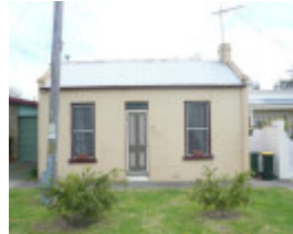
36 Mercer Street, Queenscliff
