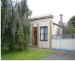
60 Mercer Street, Queenscliff
