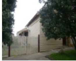
60 Mercer Street, Queenscliff
