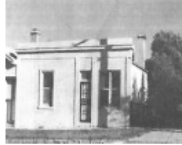
60 Mercer Street, Queenscliff
