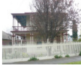
The Ridge, 68 Mercer Street, Queenscliff
