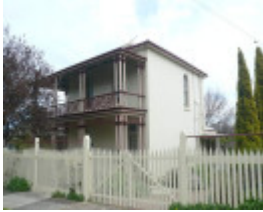
The Ridge, 68 Mercer Street, Queenscliff
