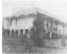
El Tambo c.1870, 80 Mercer Street, Queenscliff
