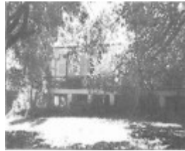
Warringah, 1981, 80 Mercer Street, Queenscliff
