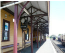
Platform of the Queenscliff Railway Station
