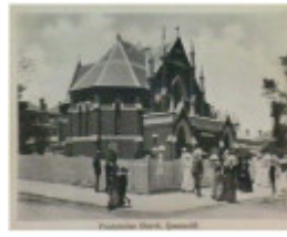
Presbyterian Church (St Andrews Uniting Church), 88-89 Hesse Street Source: State Library Victoria-undated
