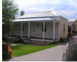
Logan Bank Cottage following recent restoration works
