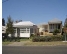
Logan Bank Cottage (left of picture) prior to recent restoration works Source: Queenscliffe Borough Council
