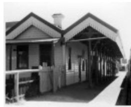
Railway Station Queenscliff c. 1981-1986 Source: State Library Victoria, Ref jc013265
