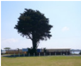
Queenscliff Railway Station, Symonds Street, Queenscliff
