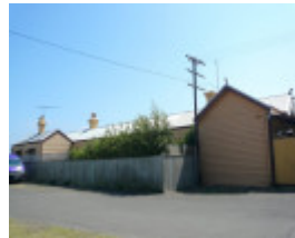
Queenscliff Railway Station, Symonds Street, Queenscliff
