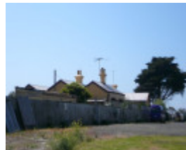
Queenscliff Railway Station, Symonds Street, Queenscliff
