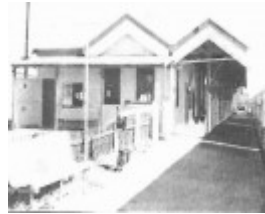
Queenscliff Railway Station, Symonds Street, Queenscliff
