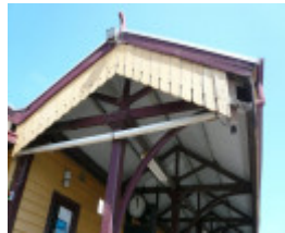
Queenscliff Railway Station, Symonds Street, Queenscliff
