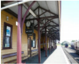
Queenscliff Railway Station, Symonds Street, Queenscliff
