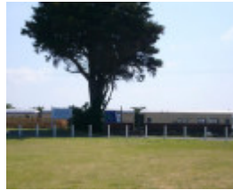
Queenscliff Railway Station, Symonds Street, Queenscliff
