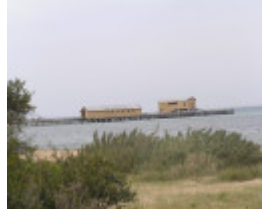
Queenscliff Pier, Shelter Shed and Lifeboat Shed, Symonds Street, Queenscliff
