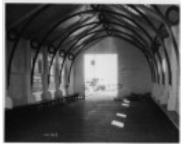
View of the interior of shelter shed on pier Queenscliff, October 1981-1986. Source: SLV (jc013262)
