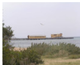
Queenscliff Pier, Shelter Shed and Lifeboat Shed, Symonds Street, Queenscliff
