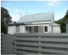
Kumala, (formerly Ripsee), 17-19 Baillieu Street, Point Lonsdale
