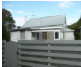
Kumala, (formerly Ripsee), 17-19 Baillieu Street, Point Lonsdale
