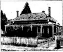
North View Villa - Ballarat Conservation Study, 1978
