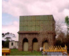
H01416 water tank werribee front view ab oct97
