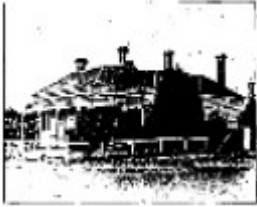
House 190 Victoria Street - Ballarat Conservation Study, 1978
