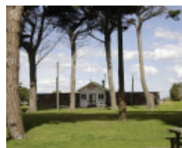
1 Tobin Drive, thought to be the 1926 shelter pavilion, former hot baths entry and change rooms building, c. 1926.
