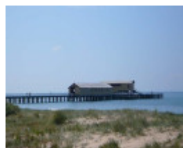
Queenscliff Pier (former Steamer Pier), with its shed and lifeboat shed, all included on the Victorian Heritage Register)
