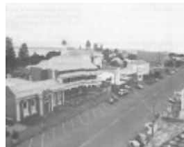
Hesse Street looking south from the Vue Grand c.1981
