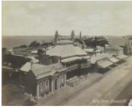
East side of Hesse Street between Hobson and Stokes Streets c. 1910. Source: SLV (a02729)
