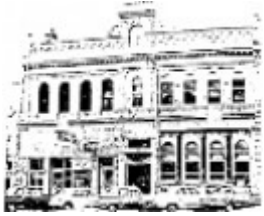
Booths Buildings - Film 1 / Frame 36 - Ballarat Conservation Study, 1978
