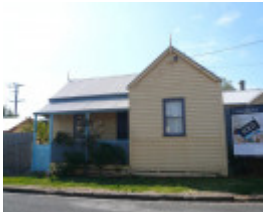
Captain Bowers Cottage, 1 St Andrews Street, Queenscliff
