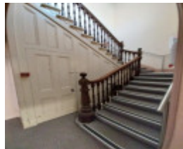
Timber joinery to internal staircase. 2023.
