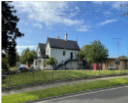
Kardinia House with bay windows and cast-iron verandahs. 2023.
