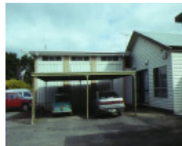
kardinia house riverview terrace belmont additions
