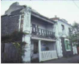
1 residence 64 capel street west melbourne front view aug1985
