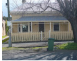
Shenfield, 96 Hesse Street, Queenscliff
