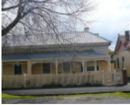
Shenfield, 96 Hesse Street, Queenscliff
