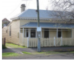
Shenfield, 96 Hesse Street, Queenscliff
