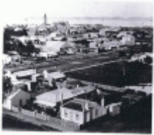
Site of former Cobb & Co. Stables, 37 Learmonth Street
