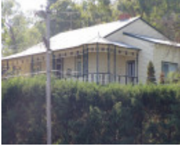
House, 3 St. Helena Road
