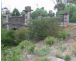
BRIDGE OVER MOONEE PONDS CREEK SOHE 2008
