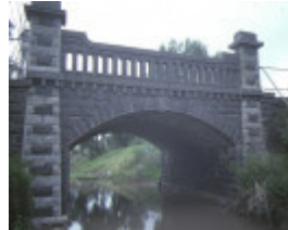
1 bridge over moonee ponds creek westmeadows front view sep1984
