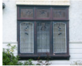
6 Waterdale Road 7 - leadlight and stained glass window.jpg
