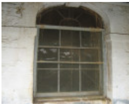
121693_former survey office_Helenslee_Heathcote_A (1).jpg
