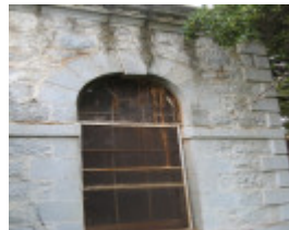
121693_former survey office_Helenslee_Heathcote_A (1).jpg
