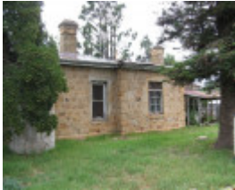
121693_former survey office_Helenslee_Heathcote_A (10).jpg
