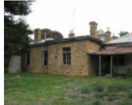
121693_former survey office_Helenslee_Heathcote_A (1).jpg
