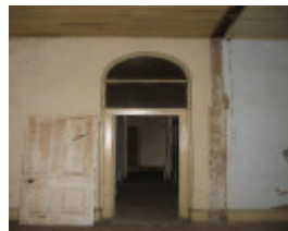
121693_former survey office_Helenslee_Heathcote_A (1).jpg
