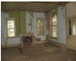
121693_former survey office_Helenslee_Heathcote_A (1).jpg
