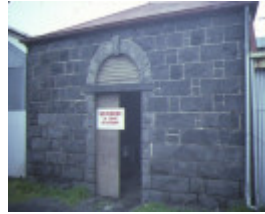
1 former morgue ann street williamstown front view sep1984
