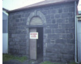
1 former morgue ann street williamstown front view sep1984
