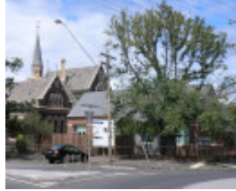
WILLIAMSTOWN PRIMARY SCHOOL NO. 1183 SOHE 2008
