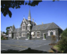
1 primary school number 1183 cecil street williamstown front view feb1993
