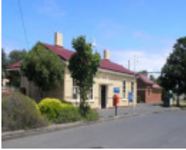
WILLIAMSTOWN RAILWAY STATION COMPLEX SOHE 2008
