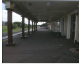
1 williamstown railway station platform canopy sept1999
