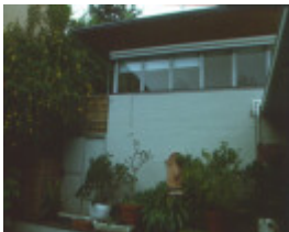
H01963 roy grounds house rear view aug01
