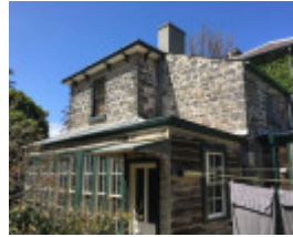
Northwest corner of bluestone fabric, showing two-storey skillion-roof portion, with the enclosed timber-framed verandah of the north elevation in foreground.
