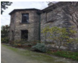
c.1882 polygonal bayed wing on left, abutting 1856-57 fabric containing two blind windows on right.
