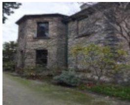
c.1882 polygonal bayed wing on left, abutting 1856-57 fabric containing two blind windows on right.
