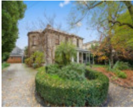
Former Presbyterian Manse from the east (Lyons Street) side. The 1991 garage building is visible at the end of the driveway on the left.
