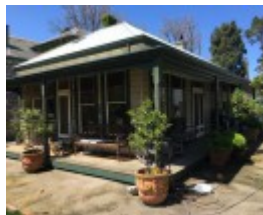
Northwest corner of mid-1980s single-storey addition.
