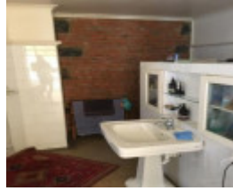
Lower-storey room, looking east at unplastered wall of original clay bricks and basalt blocks.
