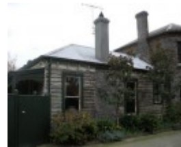
Mid-1980s single-storey addition on left, c.1882 polygonal bayed wing on right.
