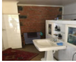
Lower-storey room, looking east at unplastered wall of original clay bricks and basalt blocks.
