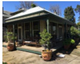
Northwest corner of mid-1980s single-storey addition.
