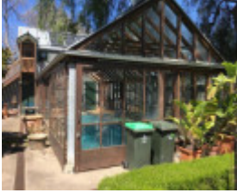
Looking south from northeast corner of 1991 pool-enclosure building, with garage beyond.
