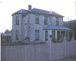
1 former presbyterian manse lyons street williamstown front view - c. early 1980s
