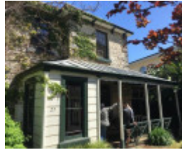
Eastern side of timber-framed verandah, with 1856-57 Former Manse above/behind.
