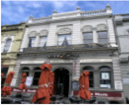
FORMER ADVERTISER BUILDING SOHE 2008
