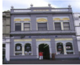
1 former advertiser building nelson place williamstown front elevation
