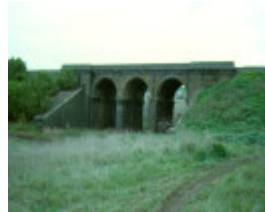
H01964 sunbury rail bridge
