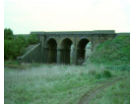
H01964 sunbury rail bridge
