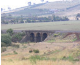
RAILWAY BRIDGE, SUNBURY HILL SOHE 2008
