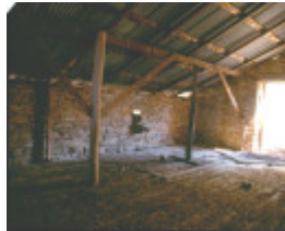
Elvezia Barn Interior 2004
