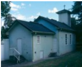
H01992 templer church hall from south east 2002
