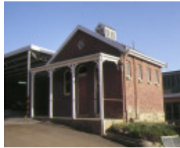
anne caudle centre building b15
