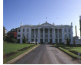
1 anne caudle centre front view of building b1 jul1992
