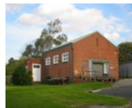
h02073 kew cottages mechanics building july2004 mz
