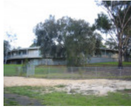
h02073 kew cottages perkin building july2004 mz
