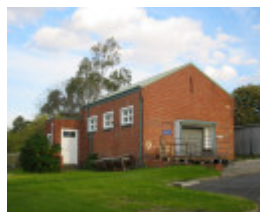
h02073 kew cottages mechanics building july2004 mz
