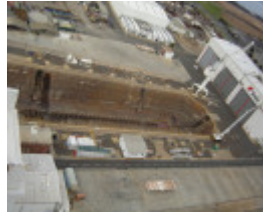
ALFRED GRAVING DOCK SOHE 2008
