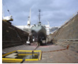
ALFRED GRAVING DOCK SOHE 2008
