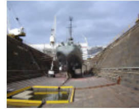
ALFRED GRAVING DOCK SOHE 2008
