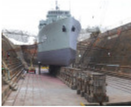
ALFRED GRAVING DOCK SOHE 2008
