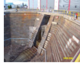
h00697 alfred graving dock williamstown dockyard williamstown steps she project 2004
