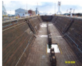
h00697 1 alfred graving dock williamstown dockyard williamstown wide view she project 2004
