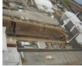
ALFRED GRAVING DOCK SOHE 2008
