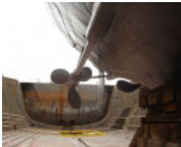
ALFRED GRAVING DOCK SOHE 2008
