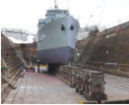
ALFRED GRAVING DOCK SOHE 2008
