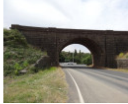
B2972 Riddells Creek rail over road bridge
