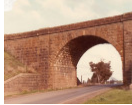
B2972 Rail Bridge over Riddell Road, Riddells Creek
