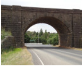
B2972 Riddells Creek rail over road bridge
