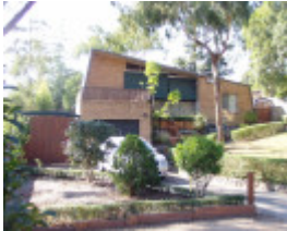
House, 209 Main Road
