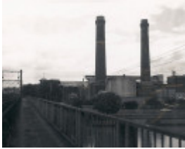
B3489 Brick Chimney Richmond Power Station
