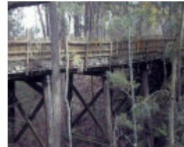
h01995 timber bridge bloomfield road crossover view of bridge she project 2003
