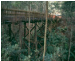
h01995 crossover bridge 2001
