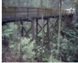
h01995 1 timber bridge bloomfield road crossover bridge she project 2003
