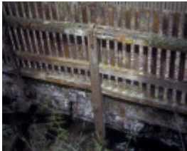
h01995 timber bridge bloomfield road crossover handrail she project 2003
