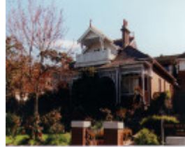
Lowana, 121 Marshall Street, constructed in 1910, is typical of the architectural character of the street.
