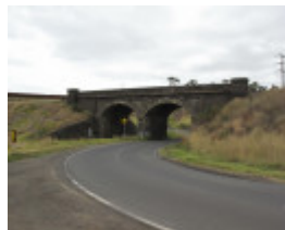
123526_Cowies Creek Rail Bridge No1_Geelong_HV_5 Feb 2010_032_resize.jpg
