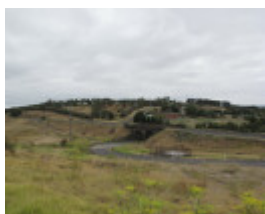
123526_Cowies Creek Rail Bridge No1_Geelong_HV_5 Feb 2010_037_resize.jpg
