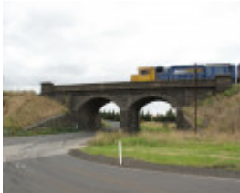
123526_Cowies Creek Rail Bridge No1_Geelong_HV_5 Feb 2010_004_resize.jpg
