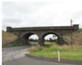
123526_Cowies Creek Rail Bridge No1_Geelong_HV_5 Feb 2010_003_resize.jpg
