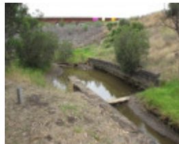
123526_Cowies Creek Rail Bridge No1_Geelong_HV_5 Feb 2010_015_resize.jpg
