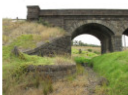
123526_Cowies Creek Rail Bridge No1_Geelong_HV_5 Feb 2010_021_resize.jpg
