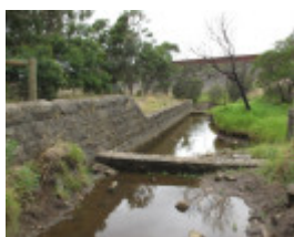
123526_Cowies Creek Rail Bridge No1_Geelong_HV_5 Feb 2010_013_resize.jpg
