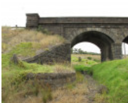
123526_Cowies Creek Rail Bridge No1_Geelong_HV_5 Feb 2010_021_resize.jpg
