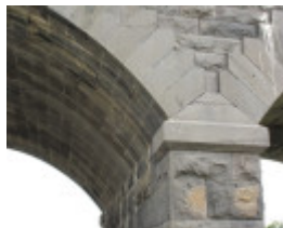
123526_Cowies Creek Rail Bridge No1_Geelong_HV_5 Feb 2010_011_resize.jpg
