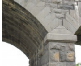
123526_Cowies Creek Rail Bridge No1_Geelong_HV_5 Feb 2010_011_resize.jpg
