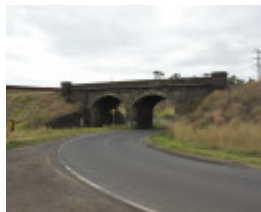
123526_Cowies Creek Rail Bridge No1_Geelong_HV_5 Feb 2010_032_resize.jpg
