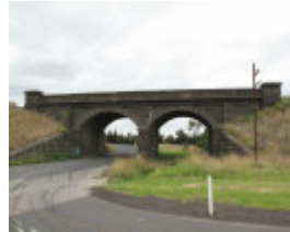
123526_Cowies Creek Rail Bridge No1_Geelong_HV_5 Feb 2010_003_resize.jpg
