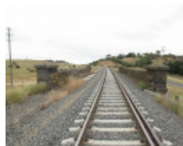
123526_Cowies Creek Rail Bridge No1_Geelong_HV_5 Feb 2010_028_resize.jpg
