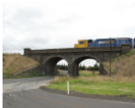
123526_Cowies Creek Rail Bridge No1_Geelong_HV_5 Feb 2010_004_resize.jpg
