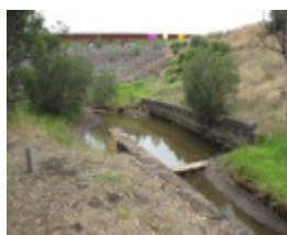
123526_Cowies Creek Rail Bridge No1_Geelong_HV_5 Feb 2010_015_resize.jpg
