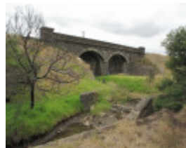
123526_Cowies Creek Rail Bridge No1_Geelong_HV_5 Feb 2010_014_resize.jpg
