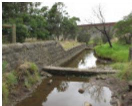
123526_Cowies Creek Rail Bridge No1_Geelong_HV_5 Feb 2010_013_resize.jpg
