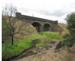
123526_Cowies Creek Rail Bridge No1_Geelong_HV_5 Feb 2010_014_resize.jpg
