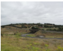
123526_Cowies Creek Rail Bridge No1_Geelong_HV_5 Feb 2010_037_resize.jpg
