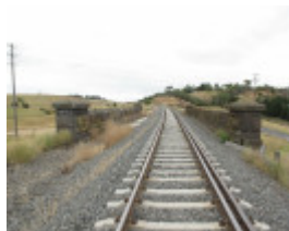
123526_Cowies Creek Rail Bridge No1_Geelong_HV_5 Feb 2010_028_resize.jpg
