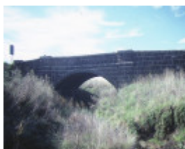
1 bridge over youls creek woolsthorpe side view jun1984
