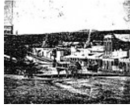
Commercial Conservation Precinct - Learmonth street looking north - 1983 Buninyong Conservation Study
