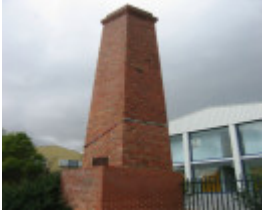
Chimney, 24 Sherbourne Road
