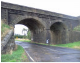
B 6394 Cowies Creek Bridge No. 1
