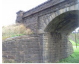
B6394 Cowies Creek Bridge No. 1 wall
