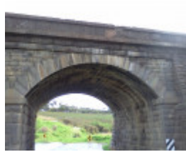
B6394 Cowies Creek Bridge No. 1 arch.
