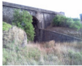
B 6395 Cowies Creek Bridge No. 2
