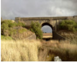
B6395 Cowies Creek Bridge No. 2
