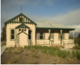
Former Shire Offices and Library, 60 Beverley Road
