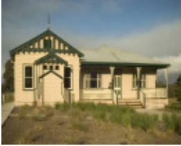
Former Shire Offices and Library, 60 Beverley Road
